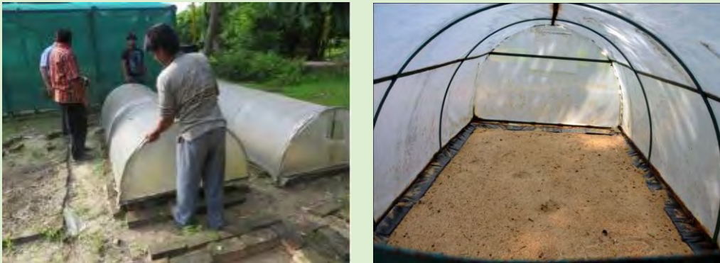
Fig 14 Domes over Hygro-pit
