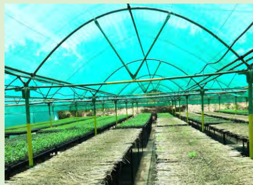
Removable shade area with galvanized steel uprights
