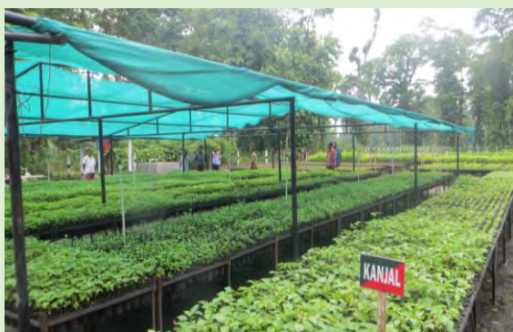
Removable shade area with galvanized steel uprights
