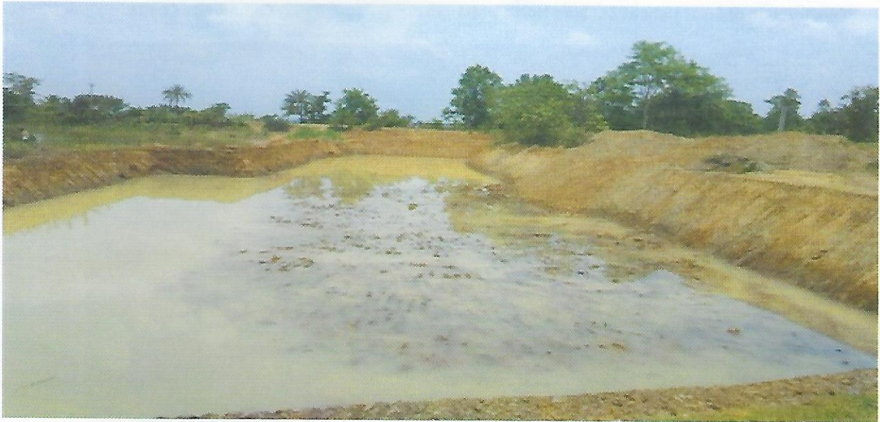
Digging of Pond-FMU- Ranibandh-JFMC- Punshya- DMU-Bankura South
