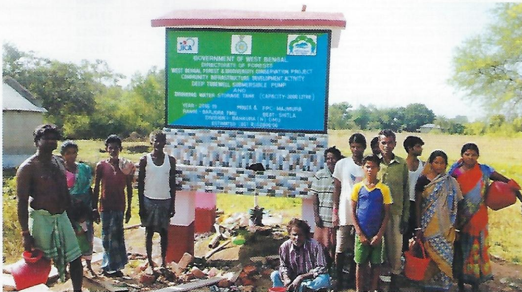
Drinking Water Storage Tank under Bankura North DMU
