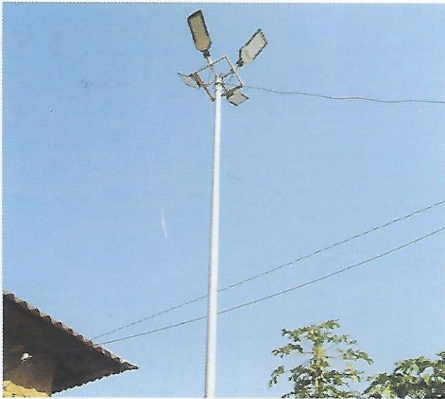
Construction of Solar Light at Bankura North DMU
