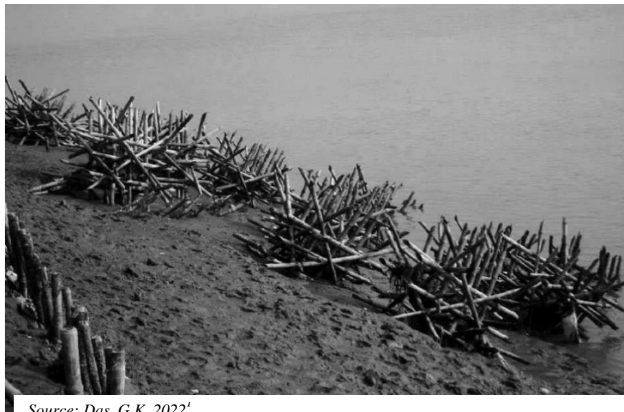
Figure 41.2 Installed Porcupine Type Structure in Sundarbans
